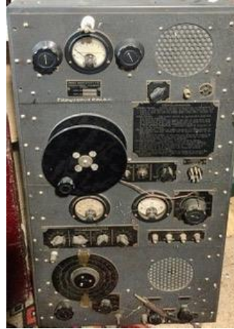
Local Broadcast Tx with SW Rx for relaying RARE
